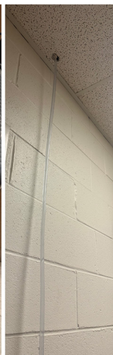
Right: Dehumidifier in the Greenville County circuit court clerk's office storage area, with a hose from the reservoir draining the water into a dehumidifier pump, then up through the ceiling tiles, and then outside.
